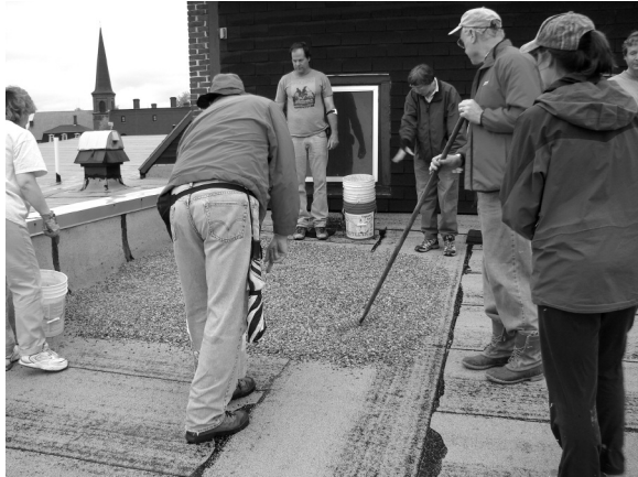
Volunteers spreading gravel on a Concord rooftop. Photo by Pam Hunt.
